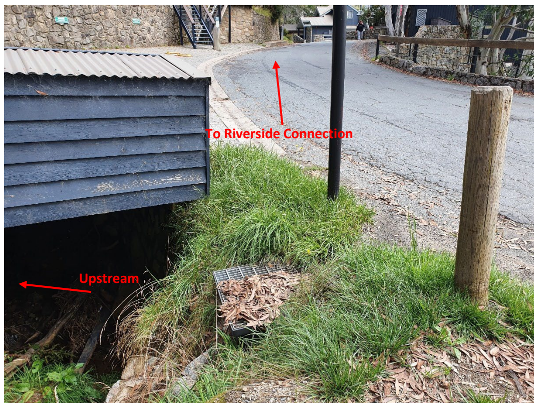
Drop inlet into minor watercourse (runs below Diggings Terrace)
