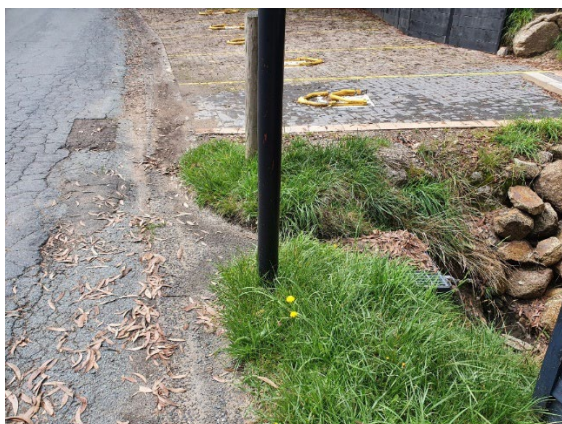
Photo A: V-drain alongside road leading into drop inlet (runs below Diggings Terrace)
